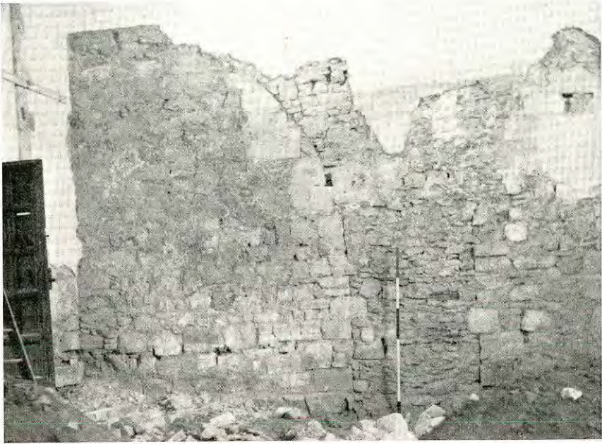
(a) Scar of Barrel Vault at S.W. end of Great Hall. Photo : Miss R. Fleming
