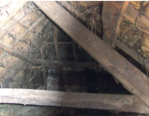
Fig. 12 Porlock, Locks Cottage, construction of earlier hipped roof still visible
