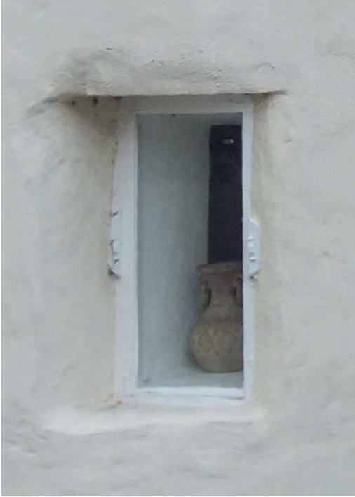
Fig. 11 Porlock, The Cottage, slit window with turnbuckles for missing shutter
