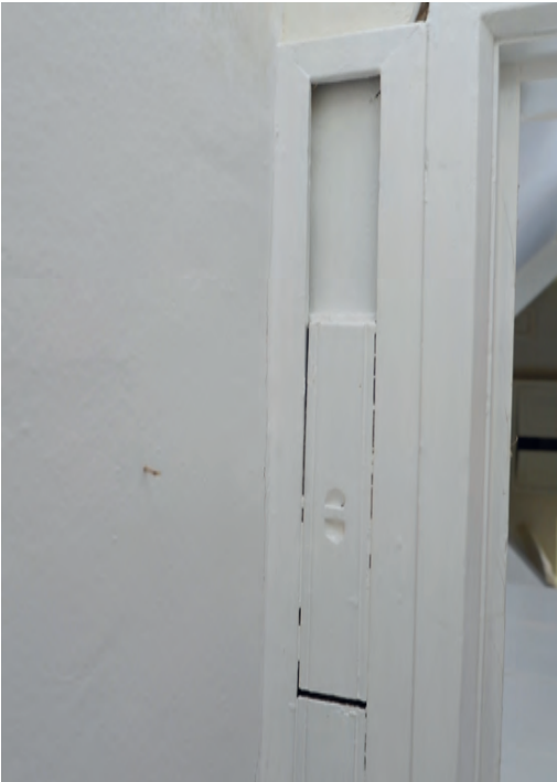
Fig. 7 Milverton, St. Mildred's, sliding ventilating door
