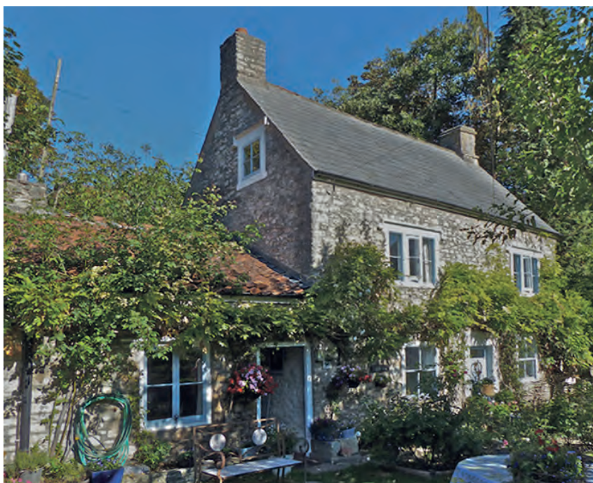
Fig. 12 Shepton Mallet, Bowlish, Wells Road, Weirside, Hood moulds over 18 th -century first-floor windows
