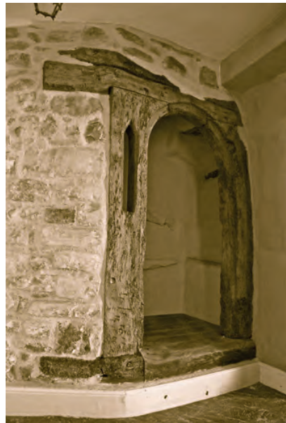
Fig. 16 Williton, Doniford, Doniford House, Door frame with pierced window at foot of solar stair turret
