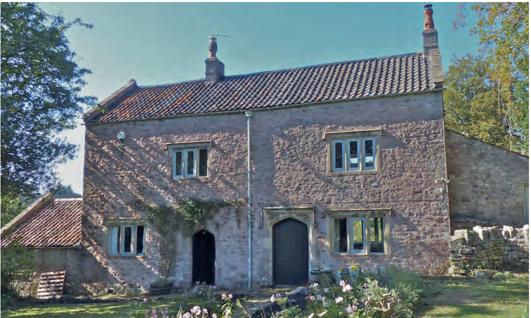
Fig. 11 Shepton Mallet, Ham, Old Manor, left-hand door is 16th century, right-hand door is 19th century. Mullioned windows inserted
