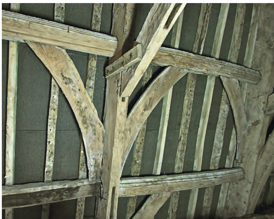
Fig. 7b Milborne Port, 14-17 High Street, Detail of the purlins and wind braces, also empty arch-brace mortices
