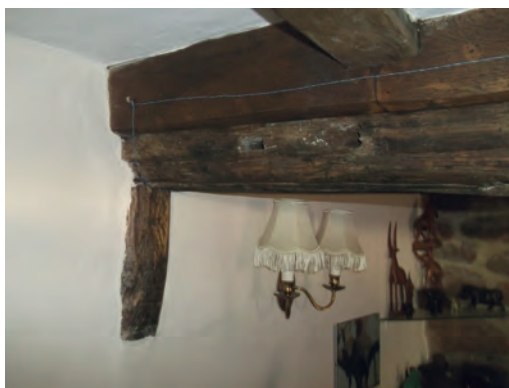
Fig. 9 Minehead, 11 Church Street, beam with roll moulding in former Hall
