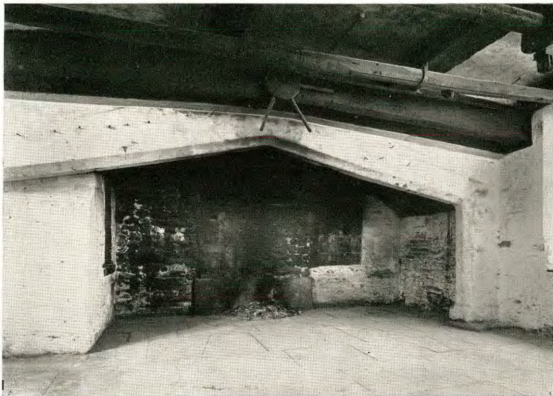
SHUTE MANOR, DEVON. The Kitchen and Fireplace, showing the Roasting Spit.
