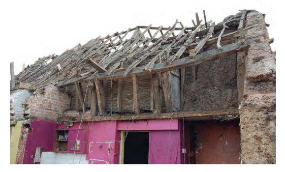
Fig. 7 Rear showing small room with door alongside cob chimney, cob gable wall, additional supports to lower purlin, and later first floor internal stud wall of reed and plaster (looking E)
