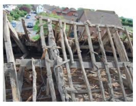
Fig. 4 Truss 1 and 2 with collars, and purlin with splayed scarf joint and dovetail joint (looking SE)
