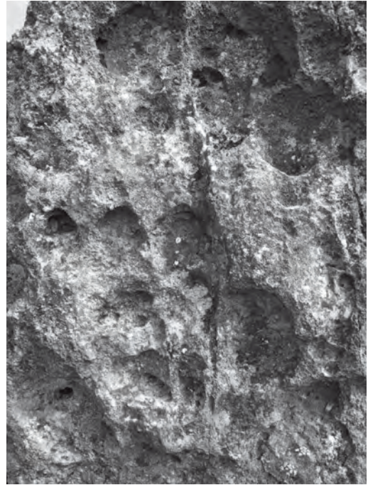
Fig. 9 Hollowing on the south face of the Yarborough standing stone
