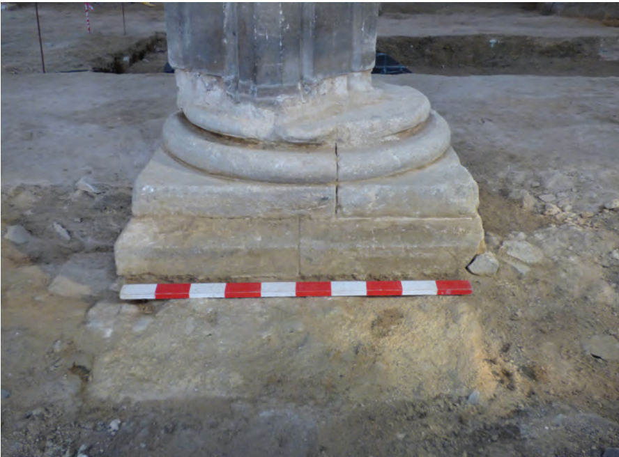
Fig. 3 Church of St John the Baptist, Glastonbury. Fifteenth-century column perched near the edge of a late Norman pier base.
