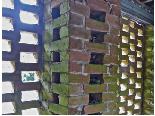
Fig. 15b Shepton Mallett, Darshill, Darshill House, Detail of brick construction of teasel-drying house
