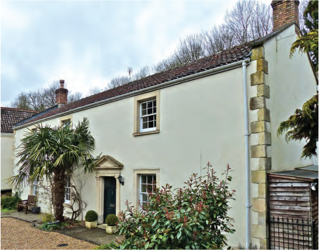
Fig. 16 Shepton Mallet, Darshill, 11 Back Lane, The Mill Masters House, Front elevation
