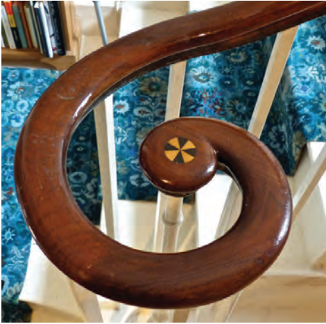
Fig. 9b Shepton Mallet, Bowlish, Coombe House, Detail of handrail at curtail step
