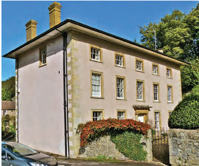
Fig. 9a Shepton Mallet, Bowlish, Coombe House, South elevation
