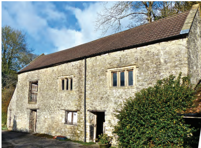
Fig. 11b Shepton Mallet, Bowlish, Park Farm House, Barn with hooded mullioned windows
