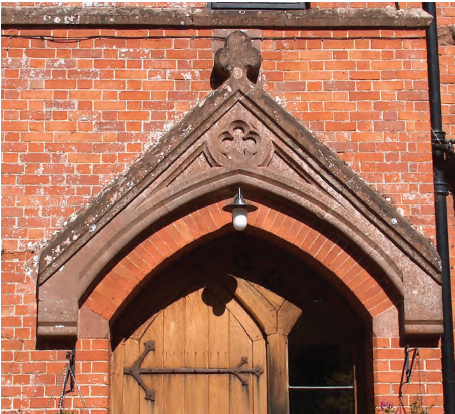
Fig. 5 The stone hood to the front door (Photo: author)
