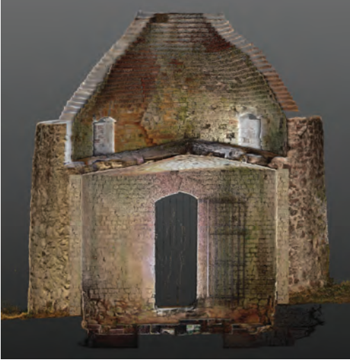
Fig. 3 Section east to west. Note the change from stonework to brickwork marking the position of the original floor. The eastern firebox has been blocked with stonework but the western only partially with roof-tiles and domestic rubbish.
