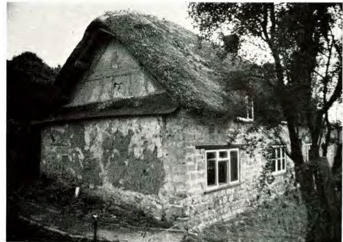
Plate VIId. Stocklinch Houses. Mannings; exterior-framed gable above cob wall.
