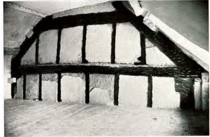
Plate VIIIb. Stocklinch Houses. Mannings; inner frame of smoke-bay (studs later).
