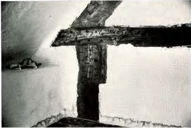
Plate VIIIa. Stocklinch Houses. Mannings; detail of post-and-truss construction.
