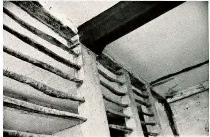
Plate VIIId. Stocklinch Houses. Mannings; partition with horizontal rods and beam with keeled stops over.
