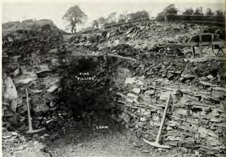
FIG. 1.—View from the S.E., showing the “fine filling,” consisting of mould and small thin pieces of lias, placed against the wall for protection.
