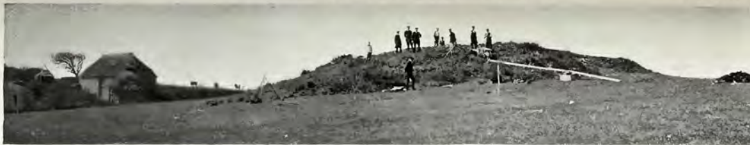
FIG. 1.—View from the S.E. on the first day of the Excavations.
