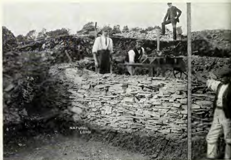
FIG. 2.—View of the south face of the Wall, showing the natural loam on which it was built.
