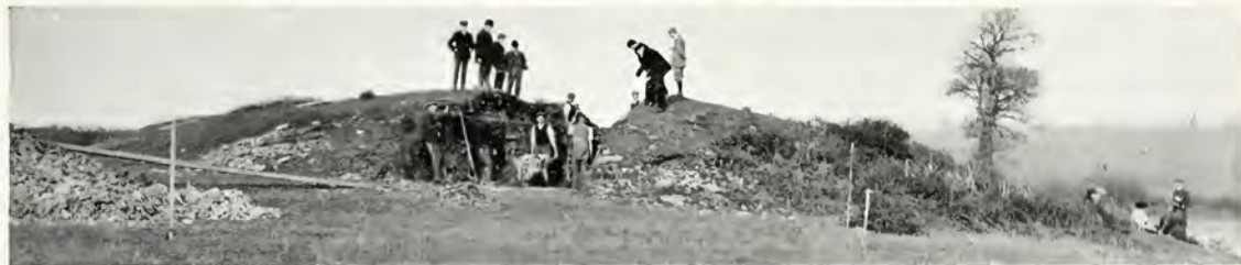
FIG. 2.—View from the W.S.W., showing the western cutting.
