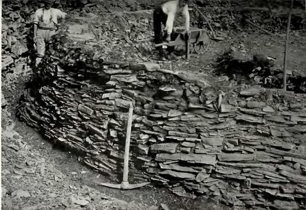
VIEW OF THE WALLED ENCLOSURE, WICK BARROW, IN ITS BEST-BUILT QUARTER ON THE W. AND N.W. ; TAKEN FROM THE W.S.W.
