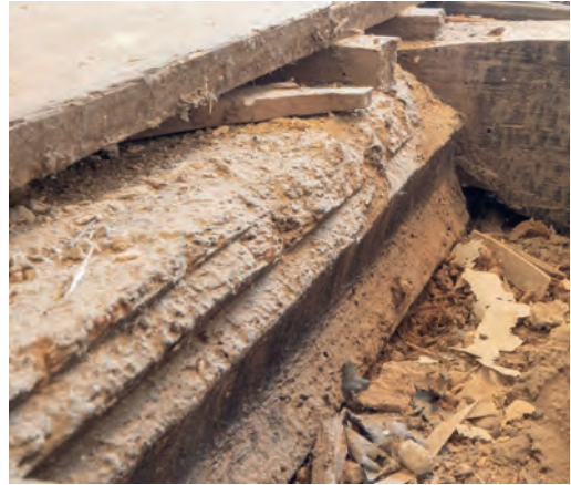
Fig. 10 Profile of assumed jetty beam b3
