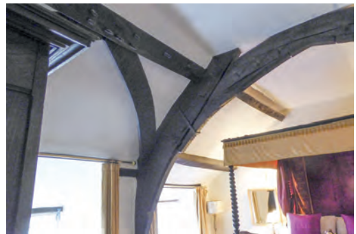
Fig. 12 Arch braced cruck truss with wind bracing
