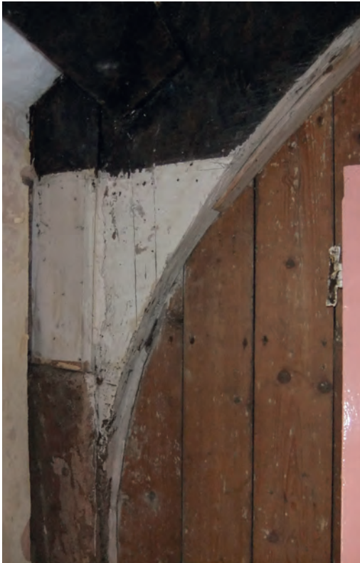
Fig. 4 True cruck (t1) truss exposed, west leg
