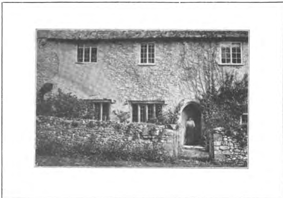
PORTION OF GATEWAY, OLDDITCH COURT.
