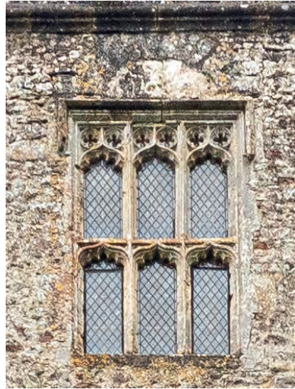
Fig. 15 Window TW2 with narrow relieving arch visible above (photo: Tony Harding)
