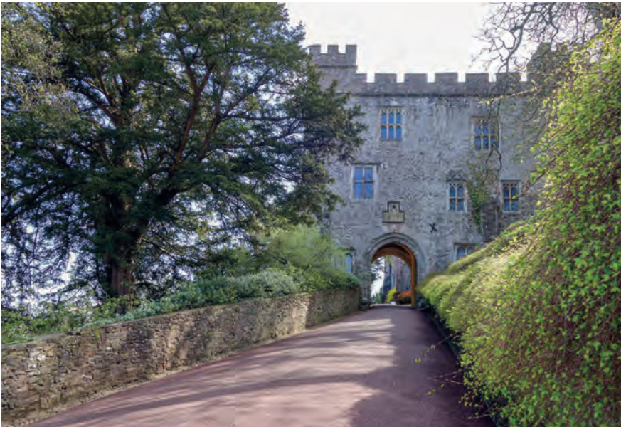
Fig. 1 Dunster Castle Gatehouse west elevation approached from the town (photo: Tony Harding)
