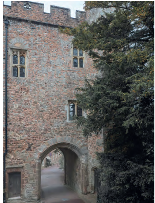
Fig. 7 The east wall of the Gatehouse
