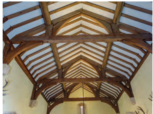
Fig. 14 The roof structure over the Tenants' Hall, 1868-70
