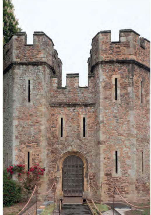
Fig. 10 The south wall with the two towers, built by Thomas Hull in 1764
