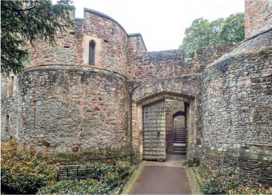
Fig. 4 The Gateway Towers with paired doors, the steps beyond lead to the Green Court (Lower Ward)
