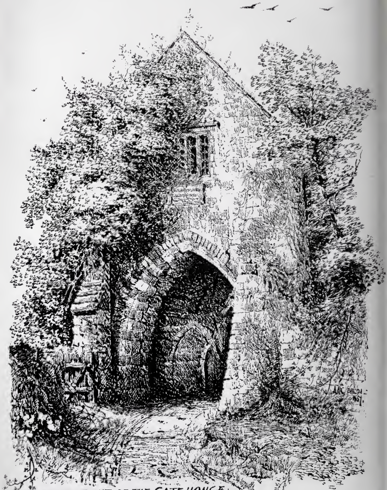
THE NORTH FRONT OF THE GATE HOUSE OLD CLEEVE ABBEY, SOMERSETSHIRE.
