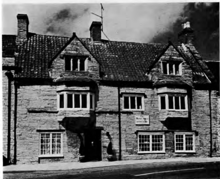
Plate 1. White House, Norton St. Philip. Medieval house modernized mid 17C; square-headed ovolo moulded windows under angled drip moulds, upper windows in dormers.
