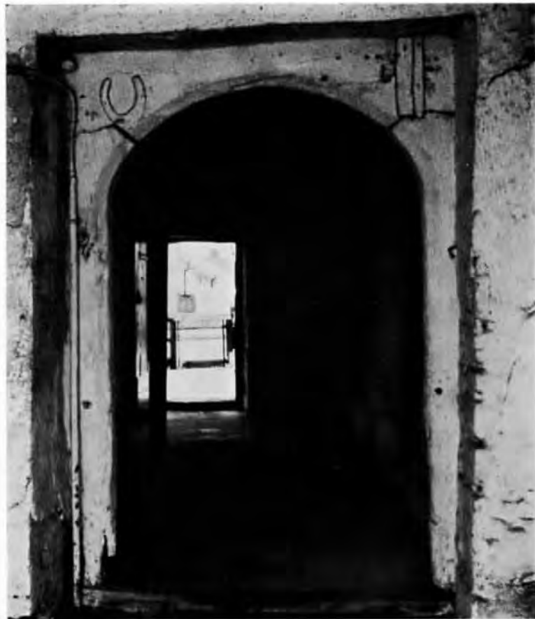
Plate 11. 115-117 Galmington Road, Taunton. Medieval three-centred doorway of the cross passage. (The house is now divided into three cottages).
