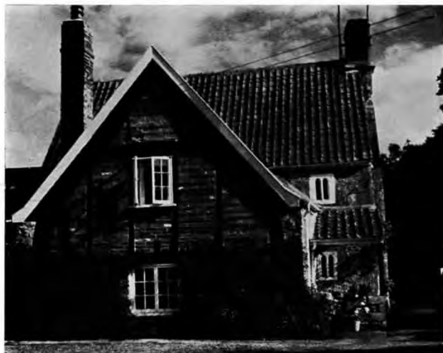
Plate 3. Craigmore, Somerton. Late 17C house with square-headed hollow mullioned windows under a stringcourse and added tall 18C wing; pediments are 18C, that on the left being an addition.
