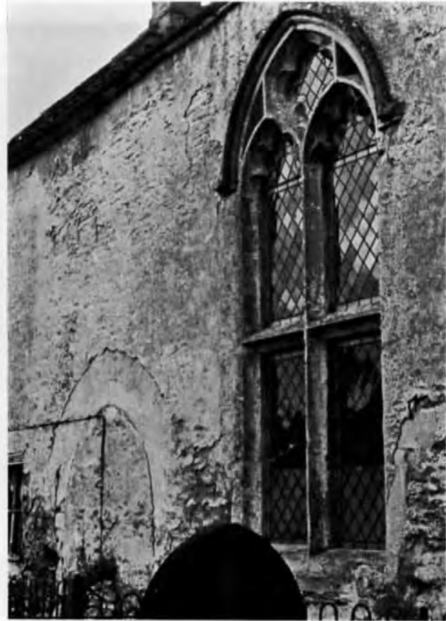
Plate 17. (right) Manor House, Croscombe. Hall window of c.1400. (Note blocked door at opposite end of cross entry to that shown in plate 9.)
