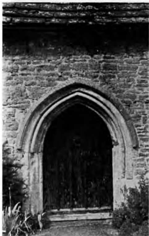
Plate 8. Wick Farmhouse, Norton St. Philip. Cross entry doorway of c.1300 with wave moulding and bulbous dripmould over two-centred head.
