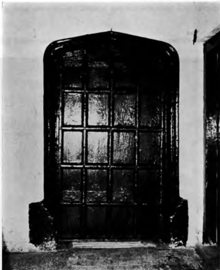
Plate 14. Hamwood Farmhouse, Trull. 17C depressed four-centred head, ovolo moulding and scroll stops.
