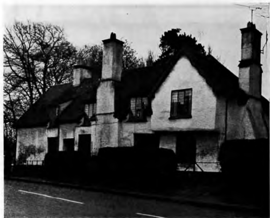
Plate 5. Burcott Manor Farmhouse, St. Cuthbert Out, Wells. Inner room of a medieval house replaced by a 17C wing giving a T plan.
