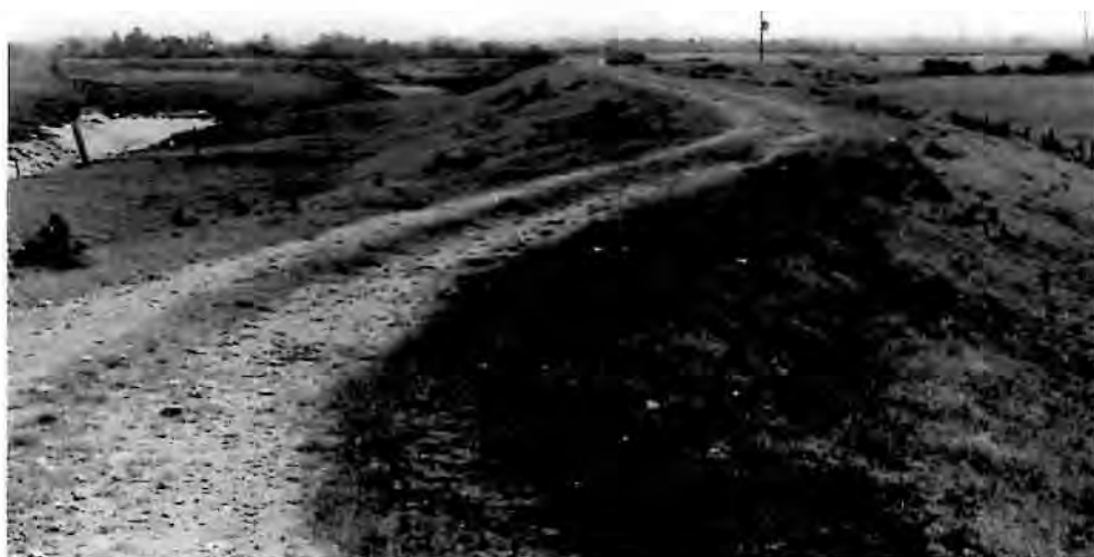
Plate 5 The newer seabank, raised and strengthened in 1990, to the northwest of New Bow, viewed toward the sluice.
