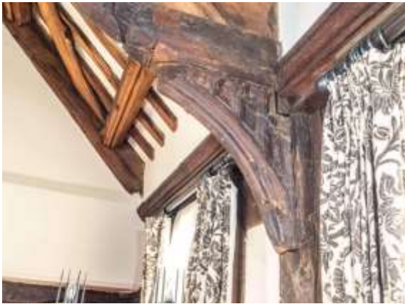
False hammer beam roof at Luttrell Arms with cusped windbracing
