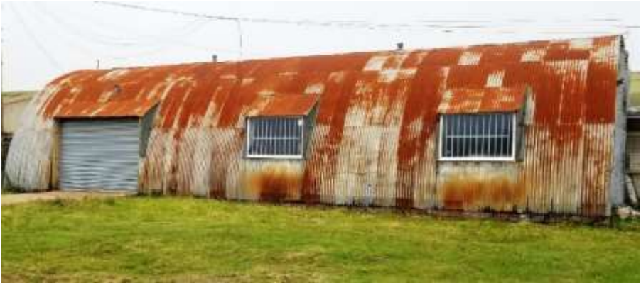
Corrugated iron Nissen hut at Dunkeswell, typical of many that were used during WW2.
