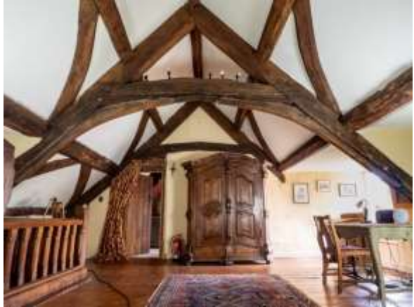
Main roof range at Lower Marsh
